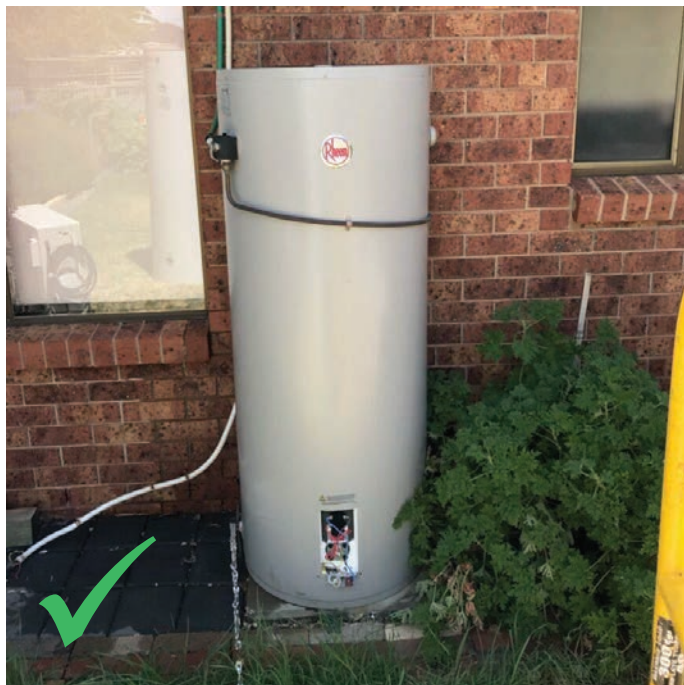
1 Shows where the old unit was installed – external or internal
