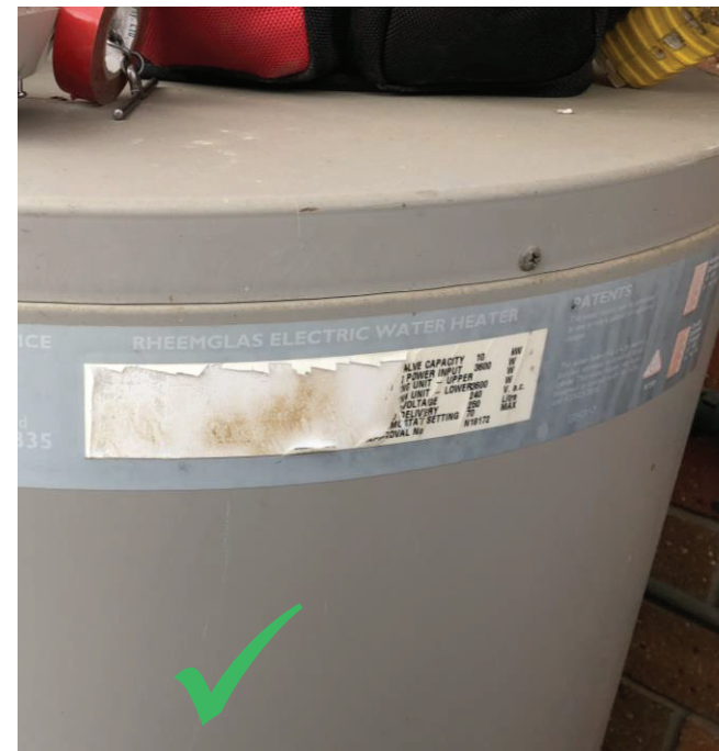
3 Shows type of old unit, weathered is OK
