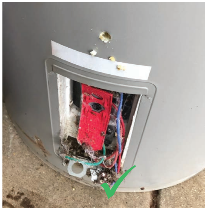
5 Clearly shows hole drilled in tank, element still in place
